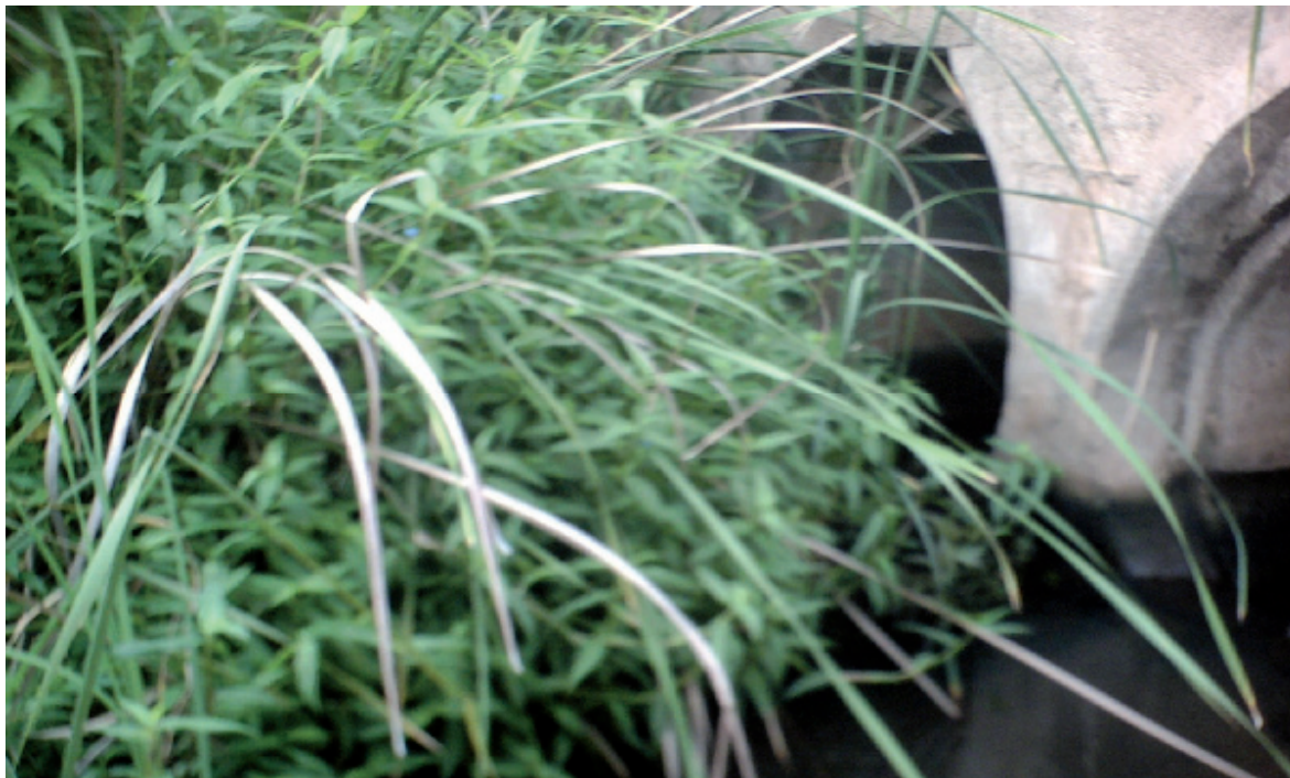
Plate 2: A concrete irrigation water drain clogged by Typha sp. Close to ‘Samawa’ main water channel
