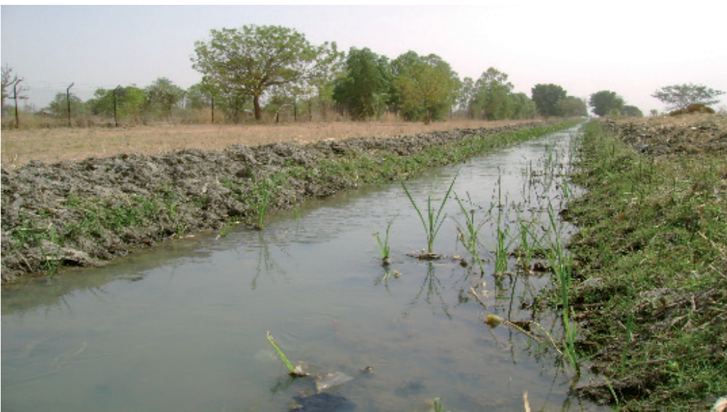
Plate 8: A canal near 'Kogin Madara' at Kura after control of Typha sp through clearing and desilting of the canal. GPS Coordinate: N11 0 ,45'33.3" E008 0 25'24.8
