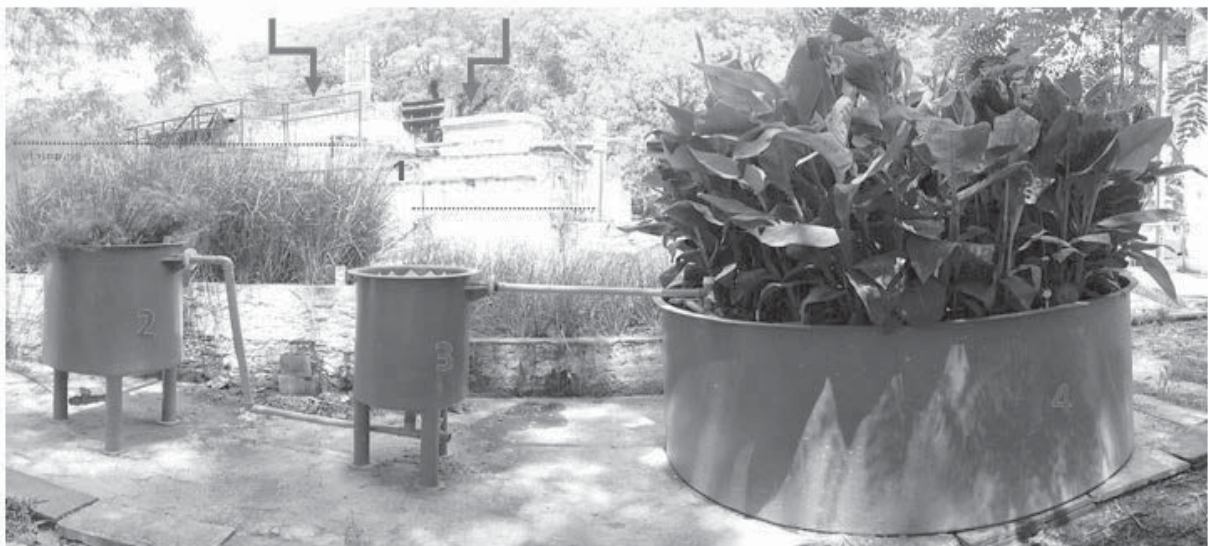
Figure 1: Treatment lines composed of hybrid constructed wetlands. Railing system (arrow left), followed by a sand box (arrow right). (1) Treatment Line I, composed of a hybrid vertical-horizontal CW; (2) surface free-flow CW with forced aeration; (3) settling unit; (4) sub-surface saturated vertical flow constructed wetland
