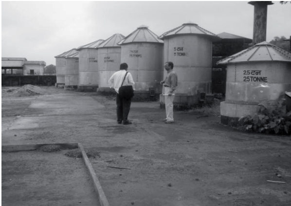
Fig. 6: Silo Storage Structures
